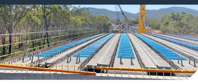
Fielders KingFlor® made with DECKFORM® steel is a permanent formwork solution suitable for concrete slabs across all types of construction, produced from 100% Australian-made BlueScope steel.
